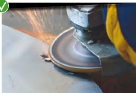
REMOVAL OF IMPERFECTIONS
